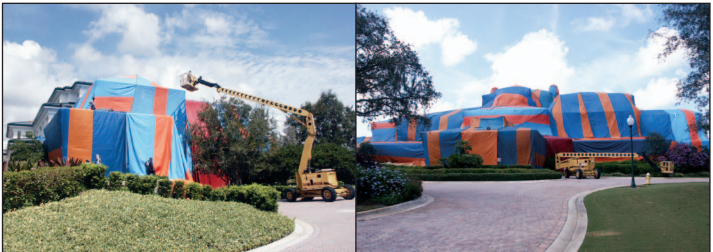
Figure 10-1. Boom lift improves safety and efficiency for tarping large structures (left and right).
