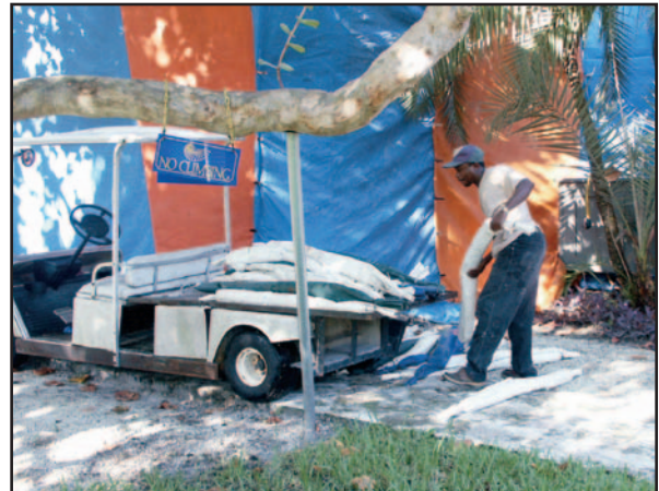
Figure 9-1. Sand snakes (and clamps) removed to free tarps for opening and removal.
