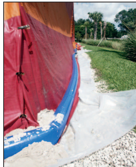
Figure 6-15. Overlapping sand snakes (left) and water snake (right). Unlike what is shown here, water snakes should be blocked in place with sand snake or heavy object.
