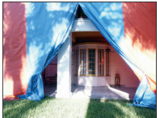
Figure 9-2. Seams are opened allowing SCBA-wearing fumigator to enter the structure and open all exterior doors to initiate Step 1 of the aeration procedure.
