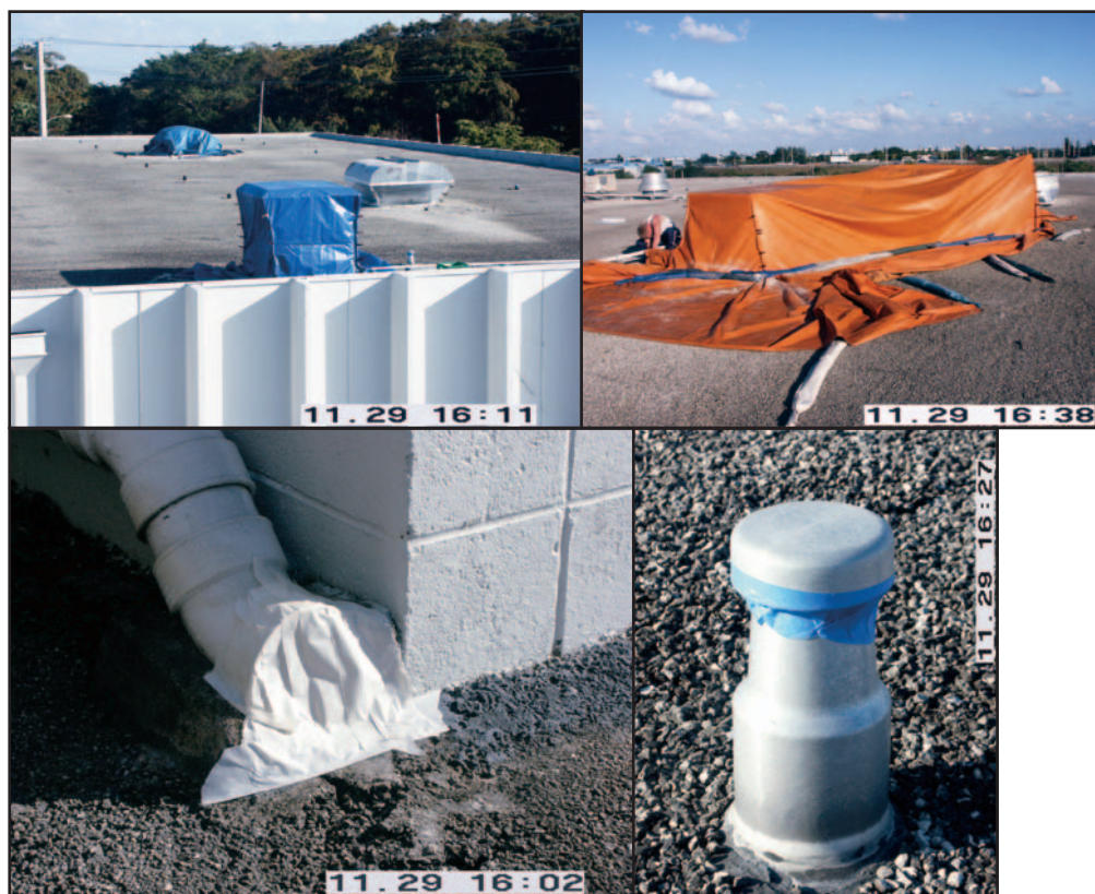
Figure 10-8. Large and strong air handlers can be covered with tarpaulins and secured with sand snakes (top left and right). Attention to detail is important to prevent unwanted leaks around downspouts and small vents (bottom left and right).
