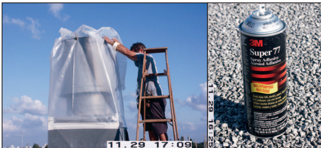
Figure 10-7. Smaller and lighter air handlers can be sealed using lightweight 4-mil polyethylene sheeting (left) secured with spray adhesive and masking or duct tape (right).
