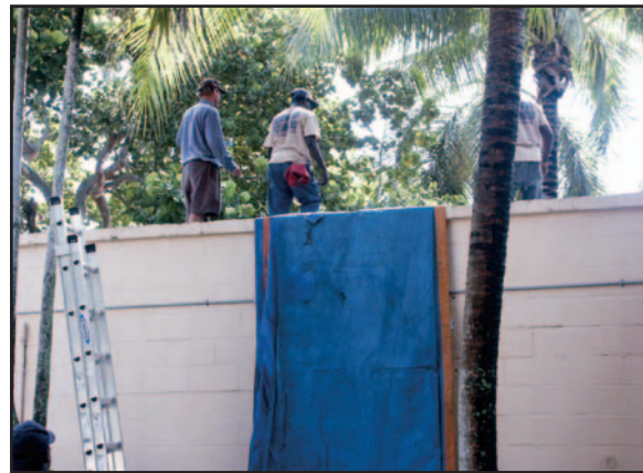
Figure 6-17. A ladder lift can safely elevate tarpaulins onto a roof (left). Balance and coordination are vital to carry tarps up a ladder (top right). Tarps are dropped down from roof (bottom right).
