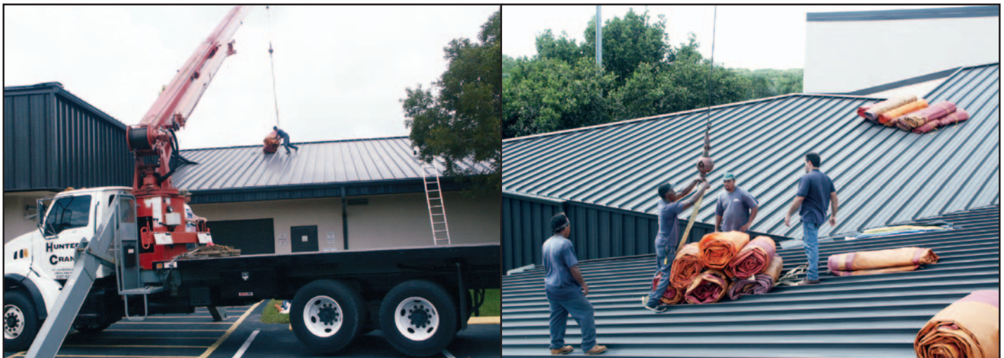
Figure 10-2. A crane can deliver tarpaulins near center of roof (left and right).
