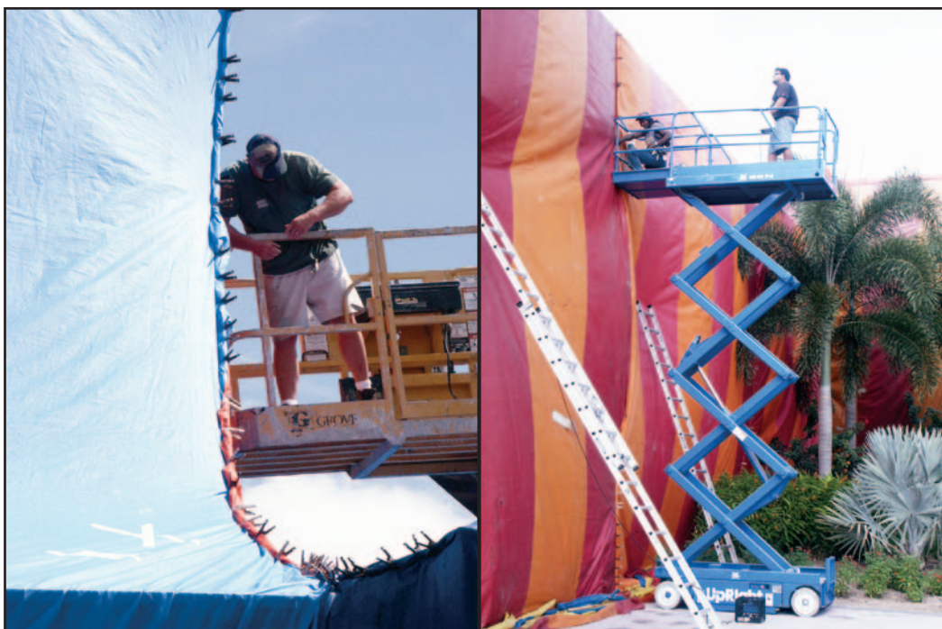
Figure 10-5. Elevated clamping from a boom lift (left) and a scissors lift (right). Note the close spacing of clamp intervals on the left.
