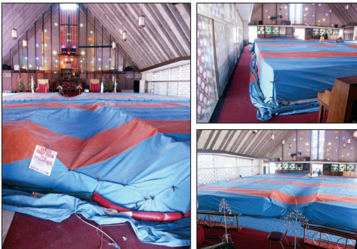
Figure 10-11. Here is a good example of fumigating a targeted part of a larger structure. All three photos show only the church pews (infested with drywood termites) were covered and snaked using standard methods. The outside of the church was secured as though the entire church was being fumigated.
