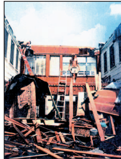
Figure 6-21. Always account for water drainage of a tarped structure. The courtyard roof of this Florida building filled with water after a heavy rainstorm and collapsed.
