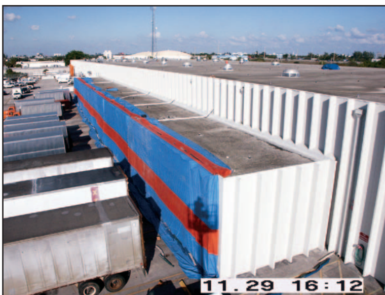
Figure 10-6. For this warehouse fumigation, tarpaulins were used to seal larger areas like delivery bays and sturdy air-handling units. Polyethylene sheeting was used for sealing smaller leaks.
