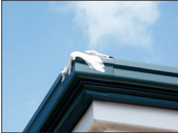
Figure 6-16. Masking tape (left) and nylon pads (right) can be used to protect tarpaulins from building corners and sharp edges.
