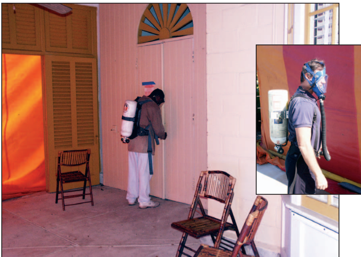
Figure 9-3. Step 1 of aeration procedure begins when the fumigator (wearing SCBA if external door is within fumigated space) has opened all operable external doors. For tape-and-seal fumigations, doors and windows must be unsealed and opened for active aeration. For tarpaulin fumigations, all operable windows should already be open during the fumigation. SCBA properly worn (inset).
