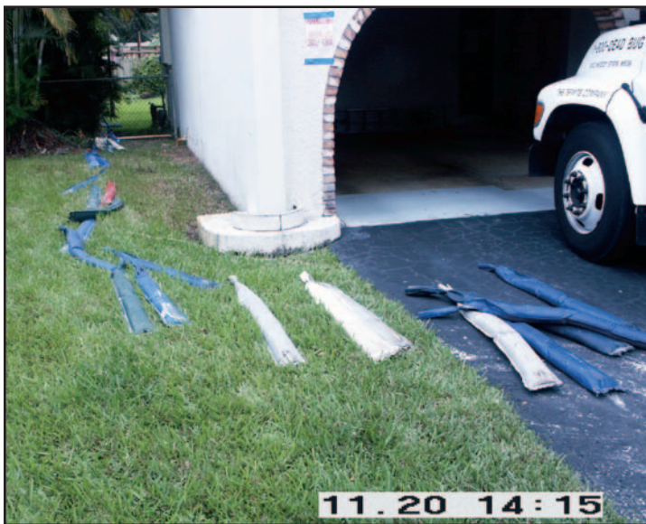
Figure 6-14. Sand snake placement before tarps are dropped.
