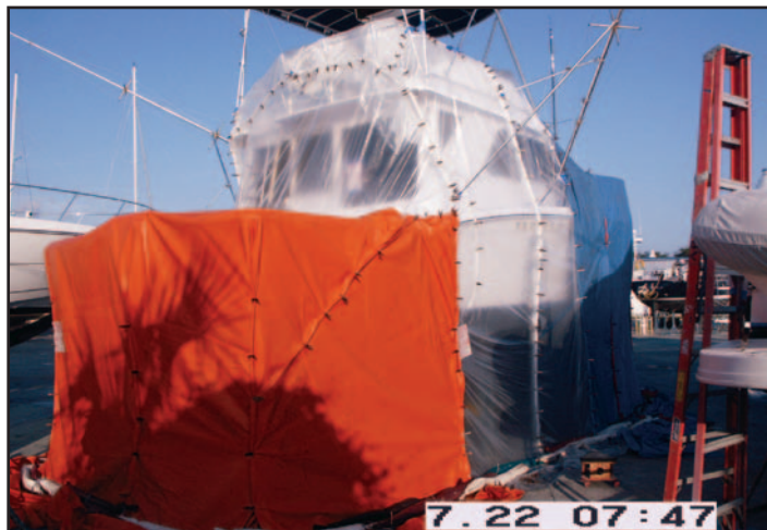
Figure 10-15. Sealing this boat in dry dock was accomplished using a combination of standard nylon/vinyl tarpaulins and 4-mil polyethylene sheeting. The poly was used to avoid damage and provide a tighter seal around the tower struts and supports.
