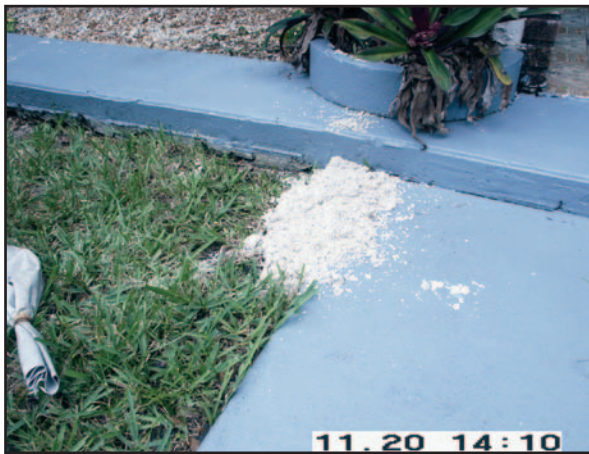
Figure 6-13. Sand placement at critical concrete/lawn junction or over a curb.
