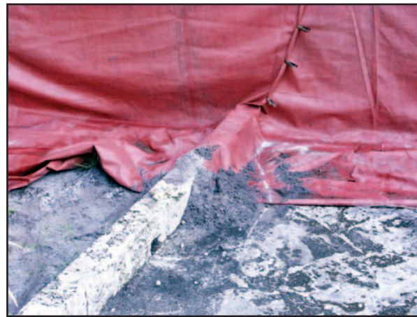
Figure 6-13. Sand placement at critical concrete/lawn junction or over a curb.
