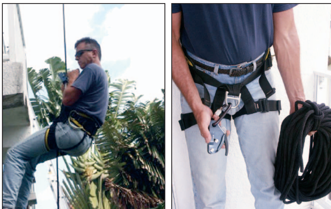
Figure 10-4. A belt slide can be used to access vertical or steep sections of tall buildings. Photos: M. Weinberg.
