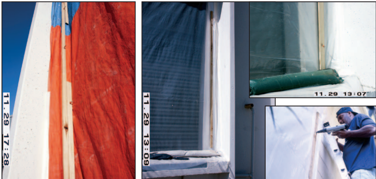
Figure 10-9. Furring strips were nailed into concrete walls (left) using a powder-actuated nail gun to support tarpaulin or 6-mil polyethylene sheeting (bottom right). Sand snakes were used on horizontal surfaces (center and top right).
