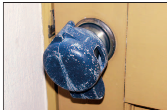
Figure 6-11. Chains with locks (top left); key block devices (top right); poles in tracks of sliding glass doors (arrow, bottom left); and clamshell key excluders (bottom right) are examples of secondary locking devices.
