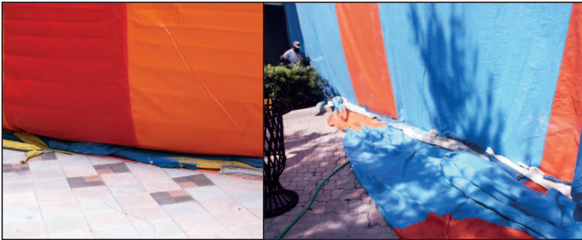
Figure 6-18. Minimal wind could pull tarp under snakes (left). Extended apron with many snakes ensures secure seal (right).
