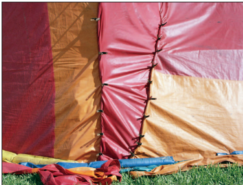
Figure 6-19. A “false” seam on the left is used to remove slack. A “hot” seam on the right joins two separate tarps.
