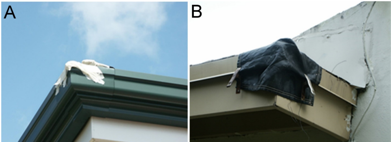
Figure 10-2. A: masking tape, and B:) nylon corner pads can be used to protect tarpaulins from building corners. (Photos: R. Scheffrahn)
