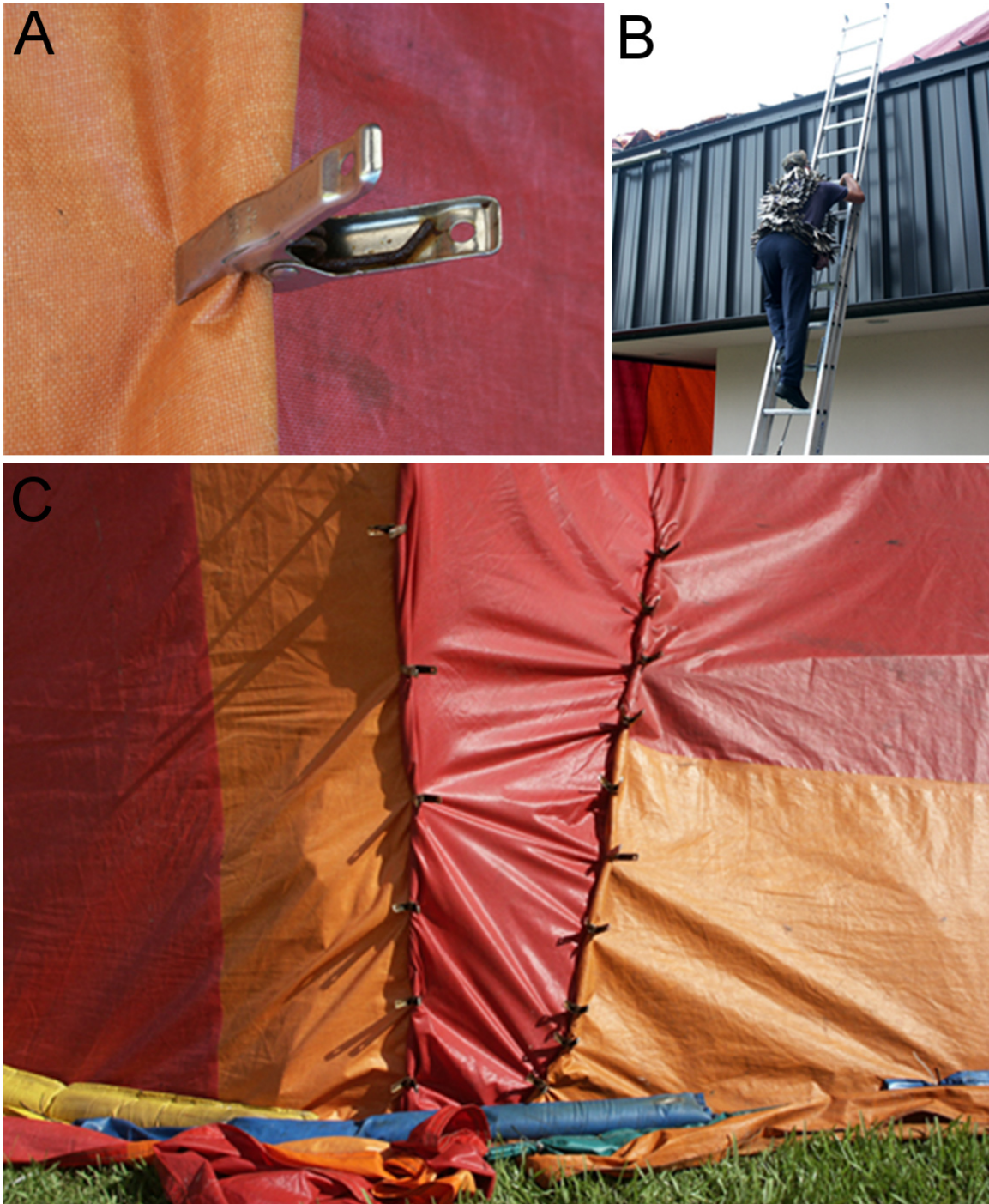
Figure 10-5. A: fumigation clamp holding rolled seam joining two tarps. B: transporting clamps on a looped rope. C: right, a "false" seam is used to remove slack; left, a "hot" seam joins two separate tarps. (Photos: R. Scheffrahn)
