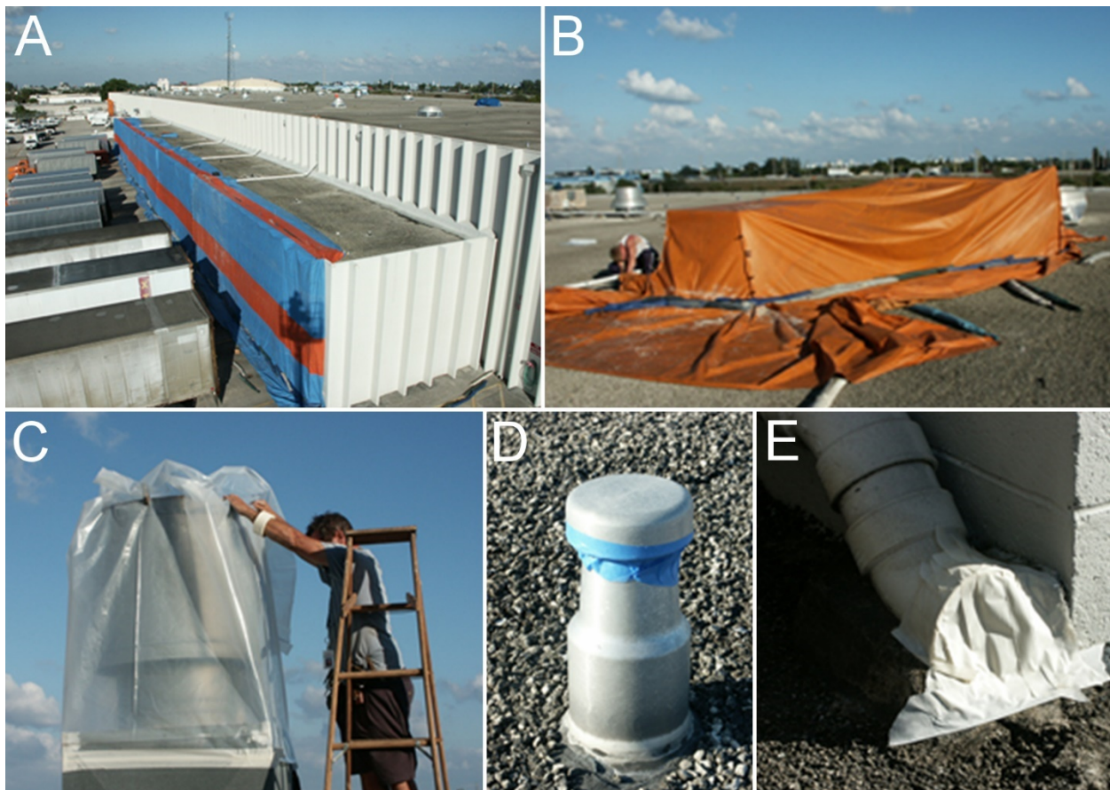
Figure 10-9. For this warehouse fumigation, tarpaulins were used to seal A: large areas like delivery bays, and B: air-handling units. C: using lightweight 4-mil polyethylene sheeting secured with spray adhesive and masking or duct tape for sealing an air handler. D: use of tape to seal gaps around small vents, and E: downspouts. (Photos: R. Scheffrahn)
