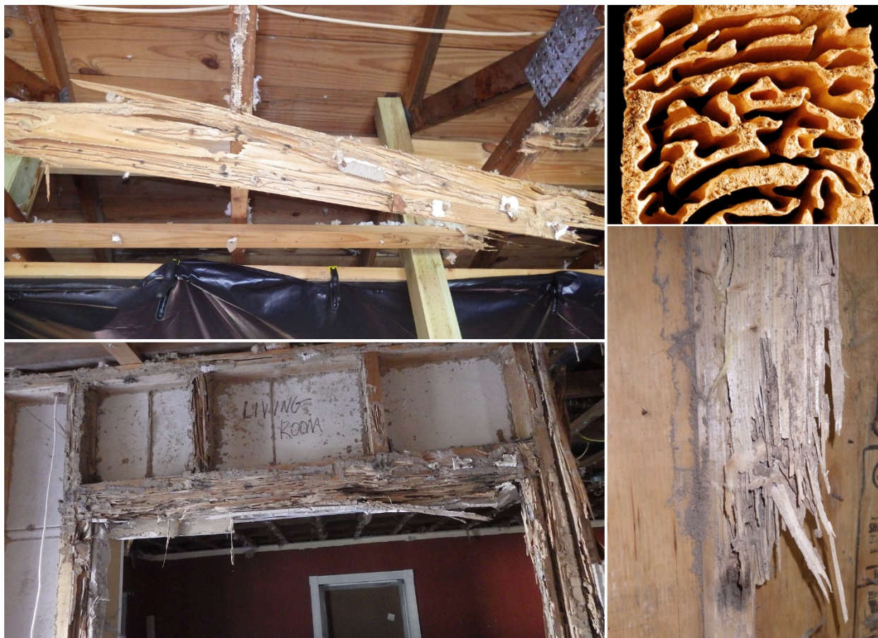
Figure 2-8. Examples of structural timber damaged by subterranean termites. The spring wood is often attacked first, and damage usually follows the grain of the wood (Photos: R. Scheffrahn, T. Chouvenec)
