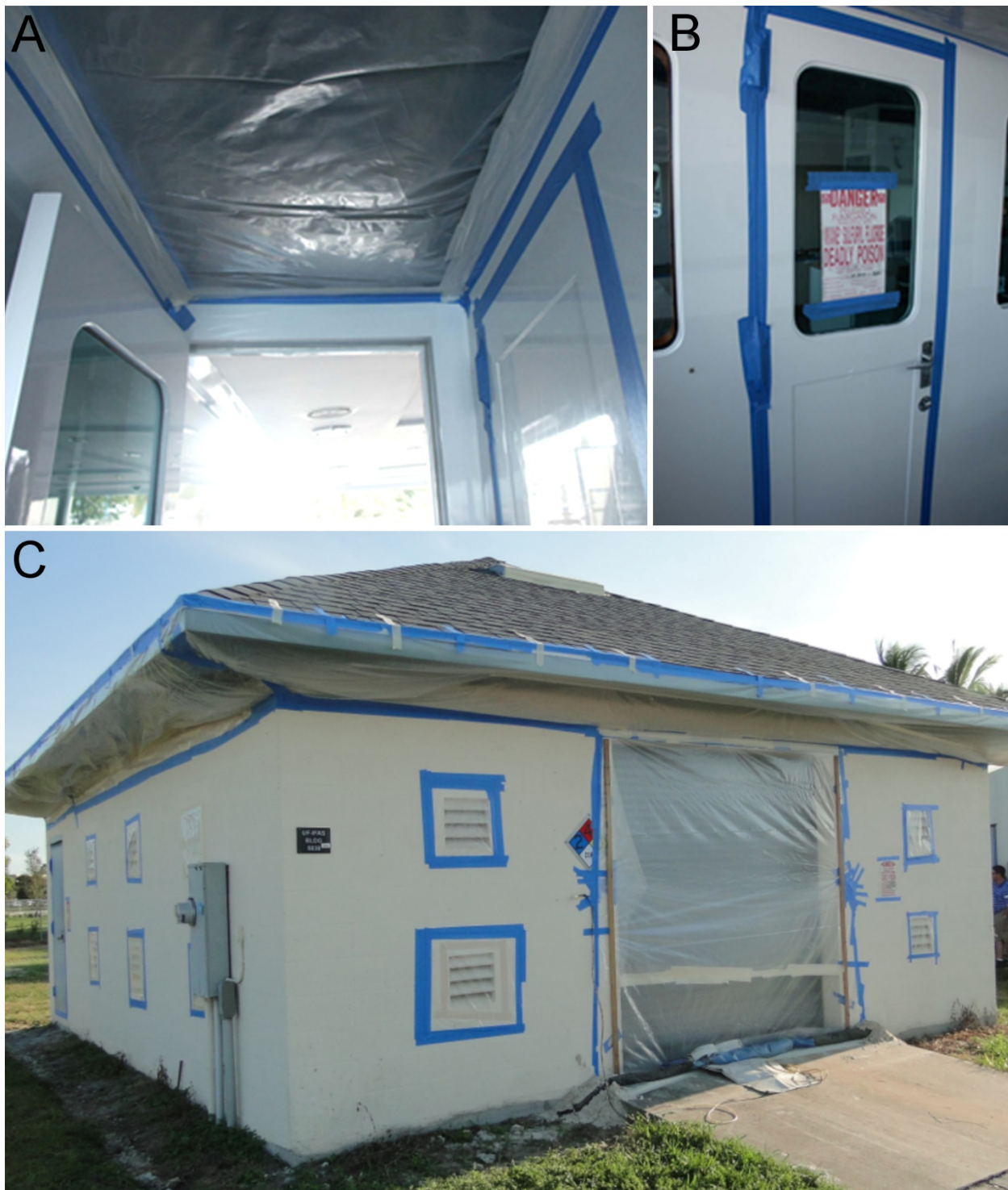
Figure 10-11. A and B: four-mil polyethylene sheeting and painter's tape is used for a gas-tight seal on a 153 ft. boat). C: tape-and-sealing fumigation a concrete block storage building. Notice four-mil polyethylene sheeting attached using painter's tape over vents, doors, and eaves to seal the building. (Photos: R. Scheffrahn)
