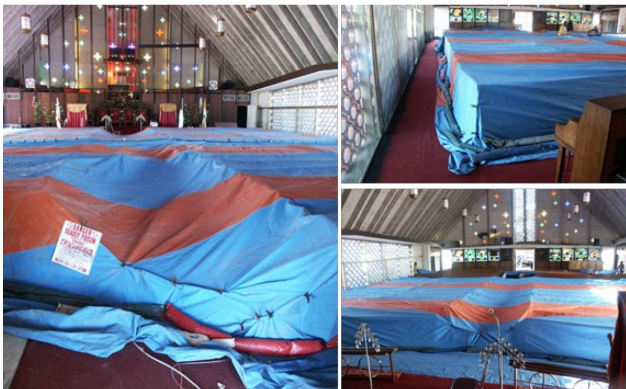
Figure 10-6. This church is a good example of fumigating targeted contents within a larger structure. Only the pews were infested with drywood termites and were tarped and snaked using standard methods (e.g., tarped stack). The church was prepared, posted, secured, and aerated as if the entire church was fumigated. Chloropicrin was only introduced into the fumigated space of the tarped pews. (Photos: R. Scheffrahn)
