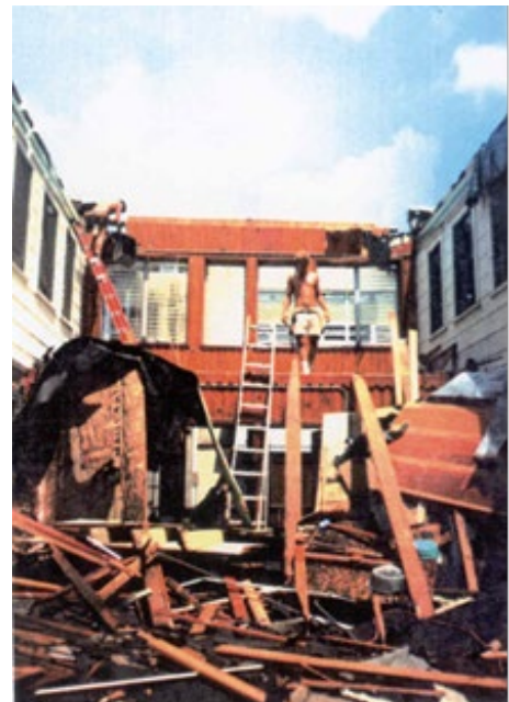
Figure 10-4. Always account for water drainage of a tarped structure. The courtyard roof of this Florida building filled with water after a heavy rainstorm and collapsed.
