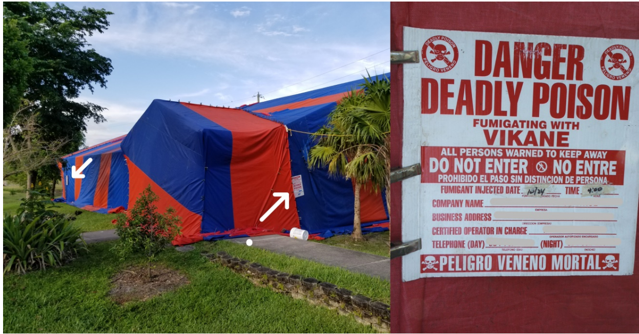
Figure 11-5. Exterior warning signs clamped to the tarpaulin. Selected warning language in Spanish is required. Clamps are a good way to ensure that signs are securely affixed to a structure. (Photos: T. Chouvinc, R. Scheffrahn)
