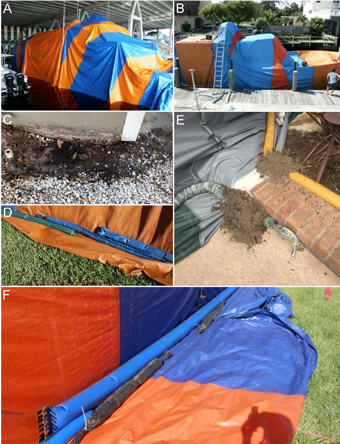
Figure 10-1. A and B: because sulfuryl fluoride is nearly insoluble in water, tarps can be dropped directly into the water. Note the depression on the bow created by the railings in the boat at the left. Provisions for storm runoff were made using a PVC pipe drain leading to a side seam. C: raking back gravel so tarps can directly contact the soil for an improved ground seal. D: overlapping snakes, E: placement of soil and tape at brick curb to seal airspaces between the tarps and the ground seal. F: water snakes correctly rolled and clamped, and blocked to prevent rolling, with additional sand snakes. (Photos: Douglas Products, R. Scheffrahn, T. Chouvenec)
